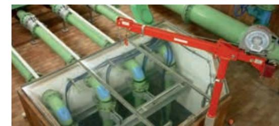
Loads, devices or pumps can be lowered and lifted using the integrated load winch.
