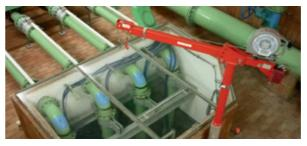
Loads, devices or pumps can be lowered and lifted using the integrated load winch.
