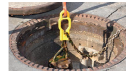
Lift a pump with chain gripper
