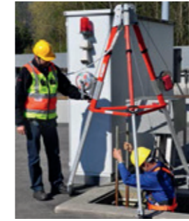
Securing person at man-hole entry with HSRG and supervising person
